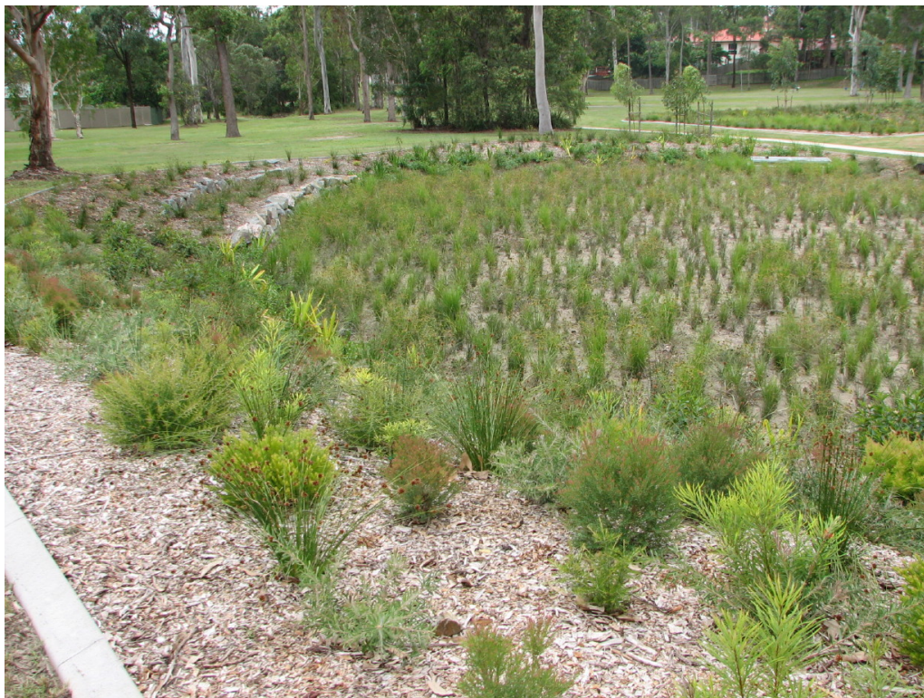
Figure 2: Typical Water Quality Bioretention Basin
